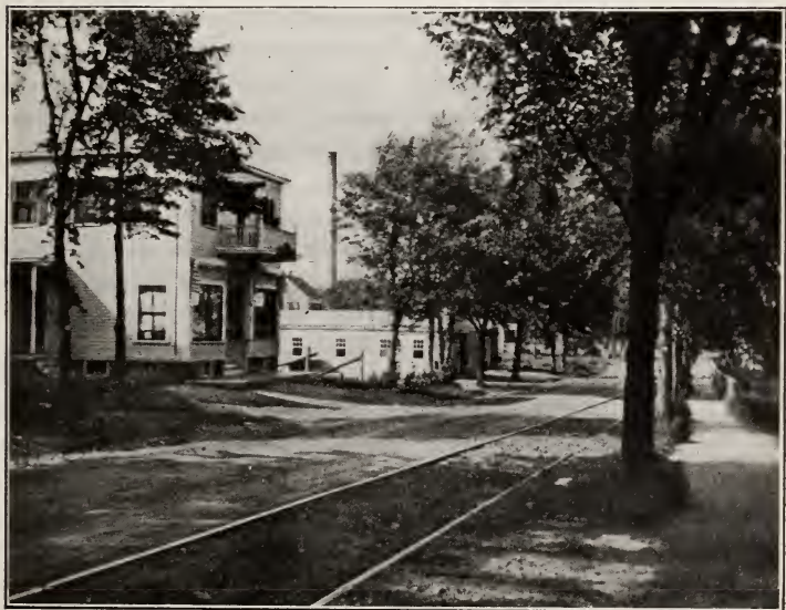
Washington Street, East Walpole. Present Width 49 Feet. Example of the Crowding which Is Piling Up Bills for the Future. Proposed Width 60 Feet, with a 10-Foot Building Line.
